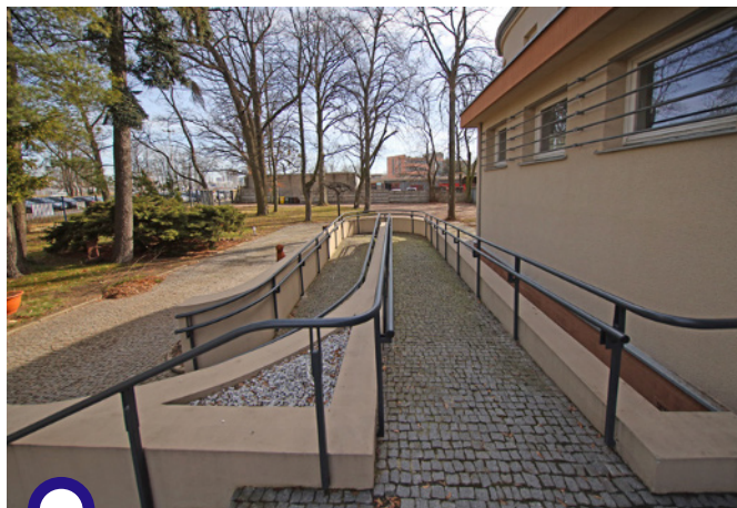
Ramps are installed at the entrance to buildings in Łódź to improve wheelchair accessibility.
